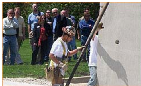
Expert erection of brick-faced architectural precast
