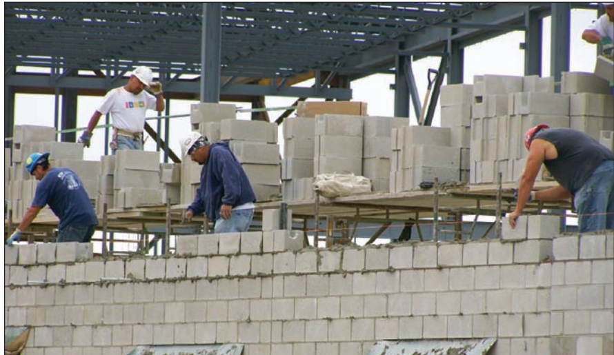
Structural masonry walls are strengthened with steel reinforcement.
