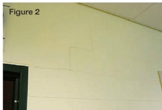
At left, a classic shrinkage crack; at right, the result of stress accumulation at corners.
