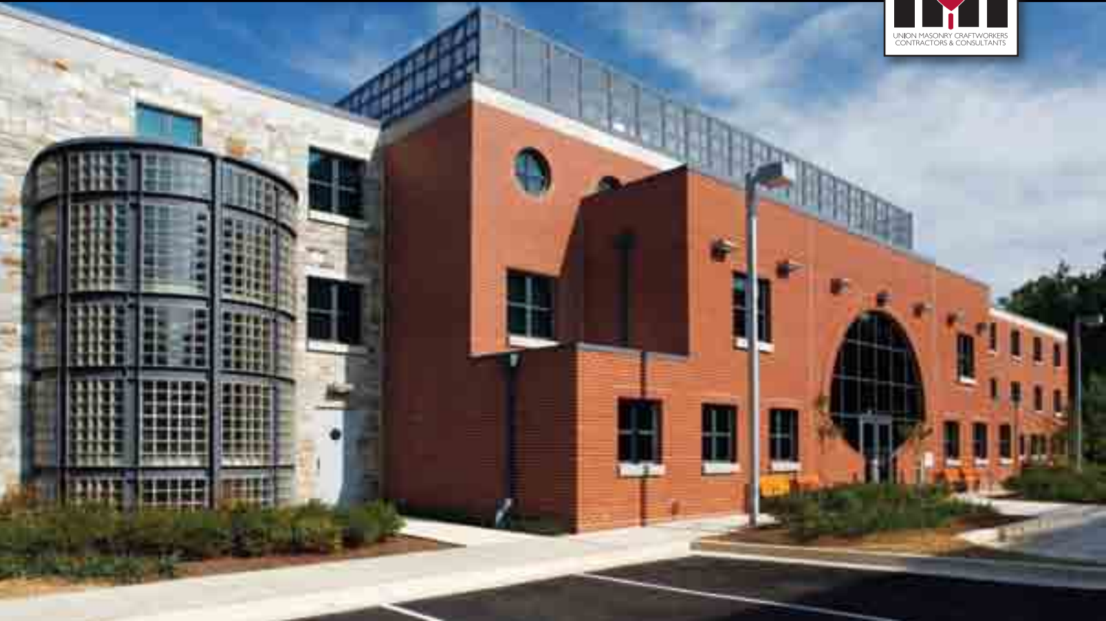
CENTER OF ATTENTION The John J. Flynn BAC/IMI International Training Center (above) in Maryland serves as the national campus of the International Masonry Institute and offers specialized training programs and events, plus education programs for designers and builders.
