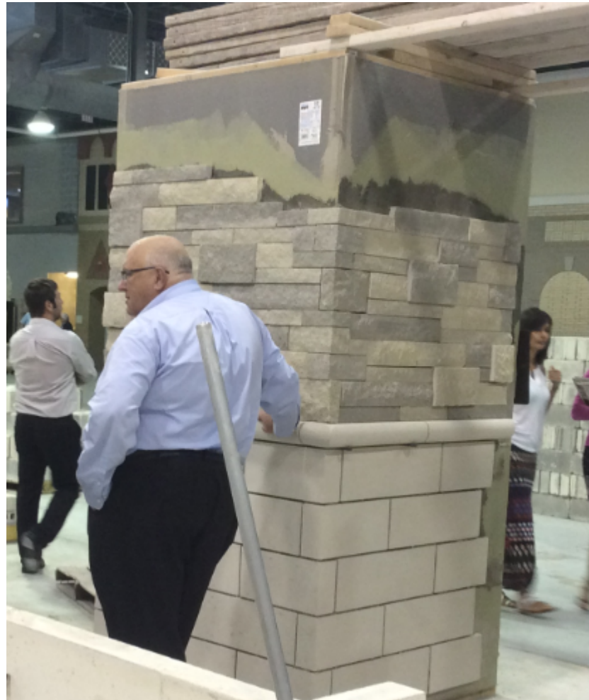
Figure 48. Wall-Section Over Continuous Rigid Insulation CMU
