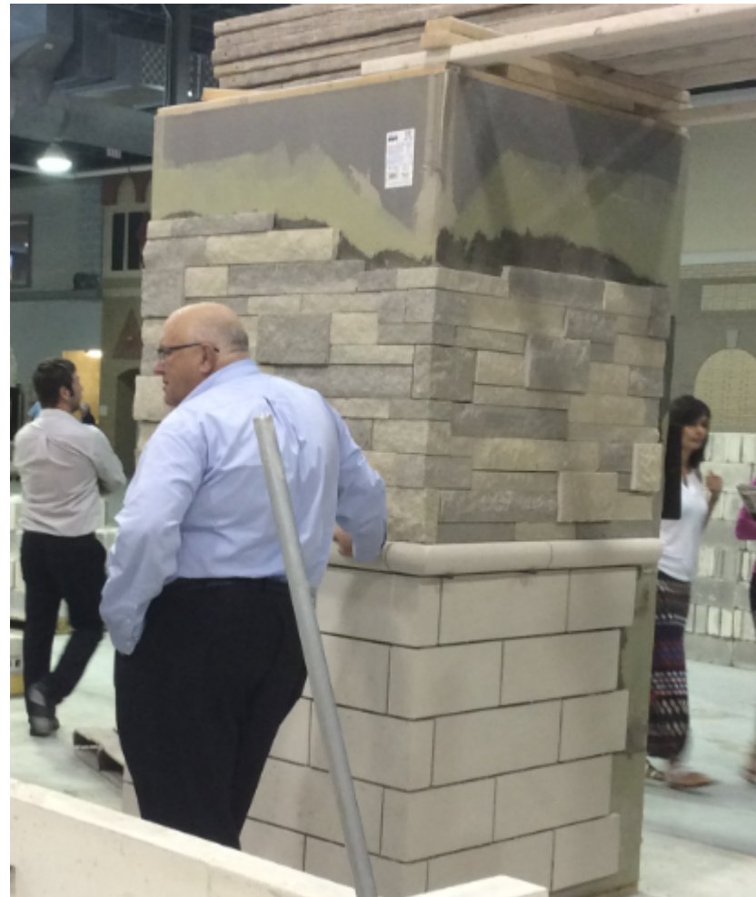
Figure 48. Wall-Section Over Continuous Rigid Insulation CMU
