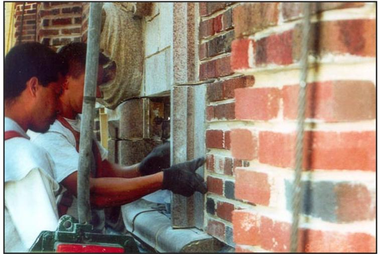
*Approximately 200 separate terra cotta pieces in 19 different profiles, shapes and sizes were replaced. Approximately 10,000 individual face bricks were also removed and replaced.*
