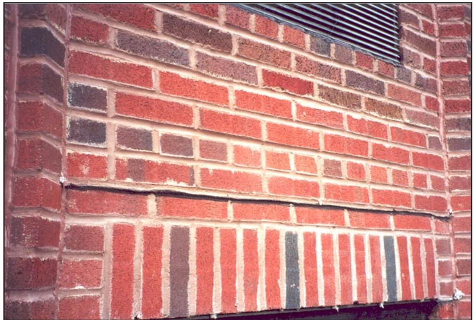
*Removal of a minimum of five brick courses both above and below the existing steel shelf angles was required ... The new face brick had to be carefully matched to the existing masonry in size, texture and, more importantly, its original “clean” color.*
