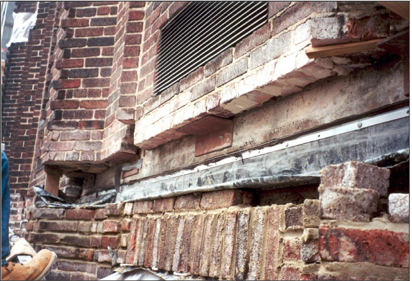
The quantity of terra cotta to be replaced was determined by carefully performing a thorough survey of each individual piece. Ultimately, over 200 separate terra cotta pieces in 19 different profiles, shapes, and sizes were replaced, either because of severe damage, or because access was needed to the structural steel supporting them.
