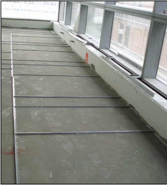
Zinc strip panels prior to Terratop matrix/binder application
