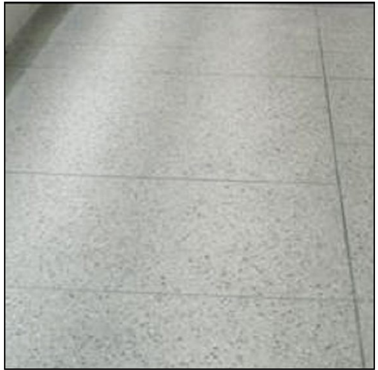
Completed Terratop Installation
