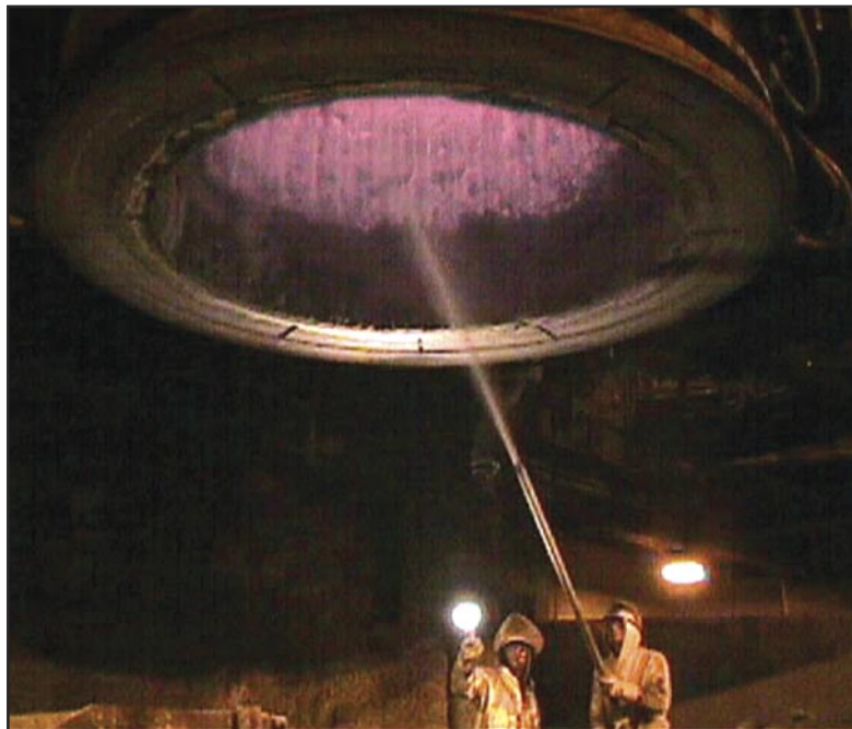
For BAC Local #4 craftworkers, daily maintenance tasks include making gunite repairs at the Vacuum De-Gasser facility (shown above) and at the Sinter Plant (below).
