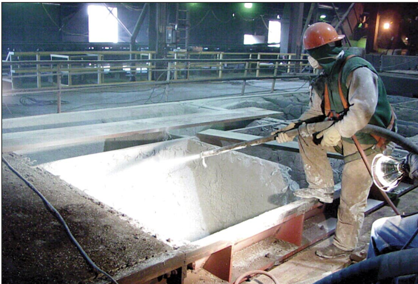
For BAC Local #4 craftworkers, daily maintenance tasks include making gunite repairs at the Vacuum De-Gasser facility (shown above) and at the Sinter Plant (below).
